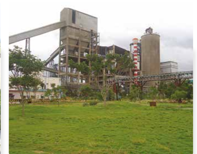
Ginigera Cement Works
